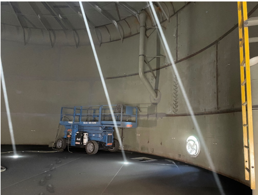
Interior of Tank 2 - Sand blasting and prepping for stripe coat
