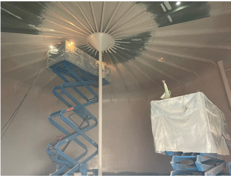
Intermediate coat - note pink tint to distinguish from top coat (white)
